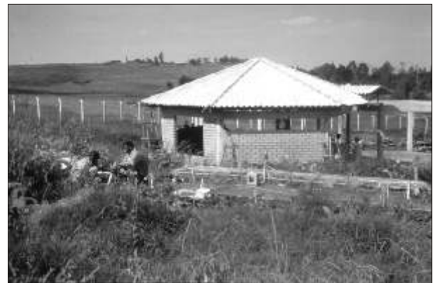
Building the classrooms in Mekaissa
